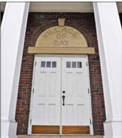
The original front entrance, which faces Dover Center Road, is no longer used.
